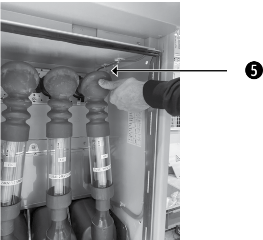
Figure 4-25: Unlock fuse holder
