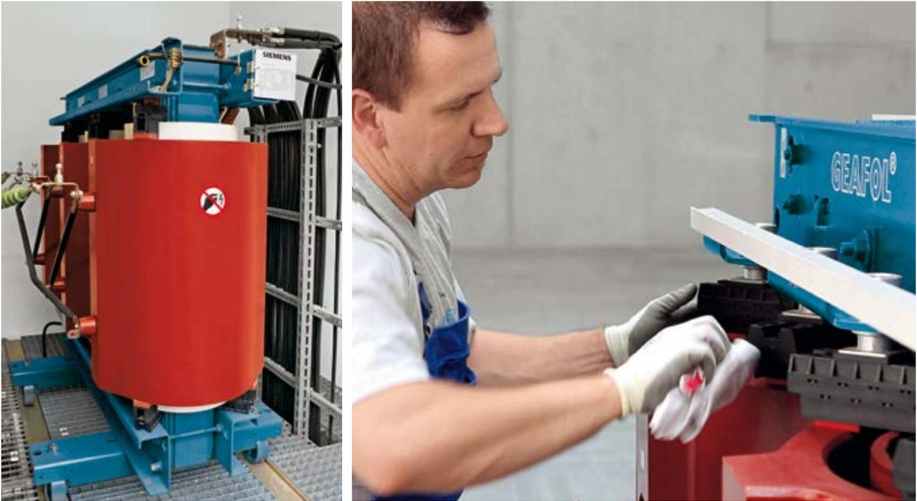
The transformer must have been cleaned and it must not contain any foreign matter (see also Installing, page 7).
